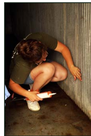
A Green Iowa AmeriCorps member caulks the walk-in cooler at Wabi Sabi Farm.
