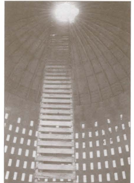
This 1950's corn crib on the farm of Arlyn and Annette Valvick revealed much hand work, including the poured cement dome.
