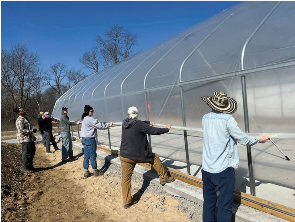
After Rosemary and Mike's greenhouse was built, volunteers from other farms helped pull the plastic and get it wired in. Community in action! (Rosemary Roelf, Singing Goat Farm, Iowa City, Iowa)
