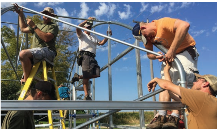
▲ From left to right: Daniel Bowser (in front of ladder), Jeremy Quigley (on ladder), Jeff Knuth, Chris Deal and Josh Nelson secure cross braces and purlines.
