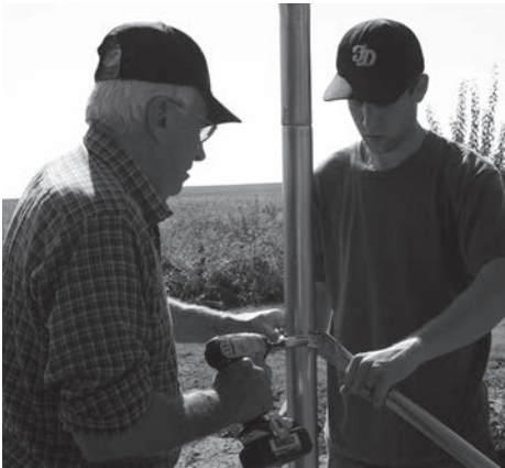
▲ Michael McNeil and Daniel Bowser close a brace band on a cross brace.
