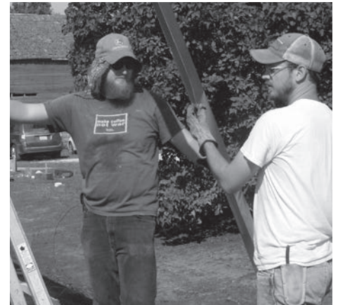
▲ Zac Couture and Josh Nelson prepare to put L-flashing on the endwall.
